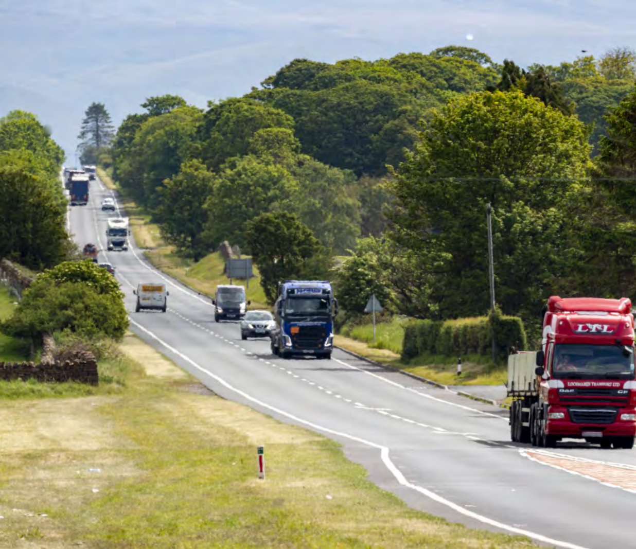
Caption: The £1 billion proposal would dual the remaining sections of A66 and improve a number of key junctions
